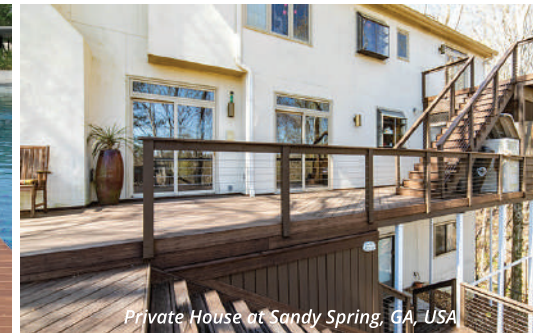
Private House at Sandy Spring, GA, USA
